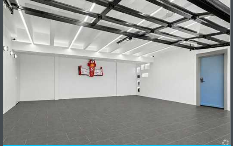
16-FOOT LINEAR LIGHTING
